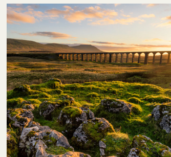
Ribblehead Viaduct Find out more
