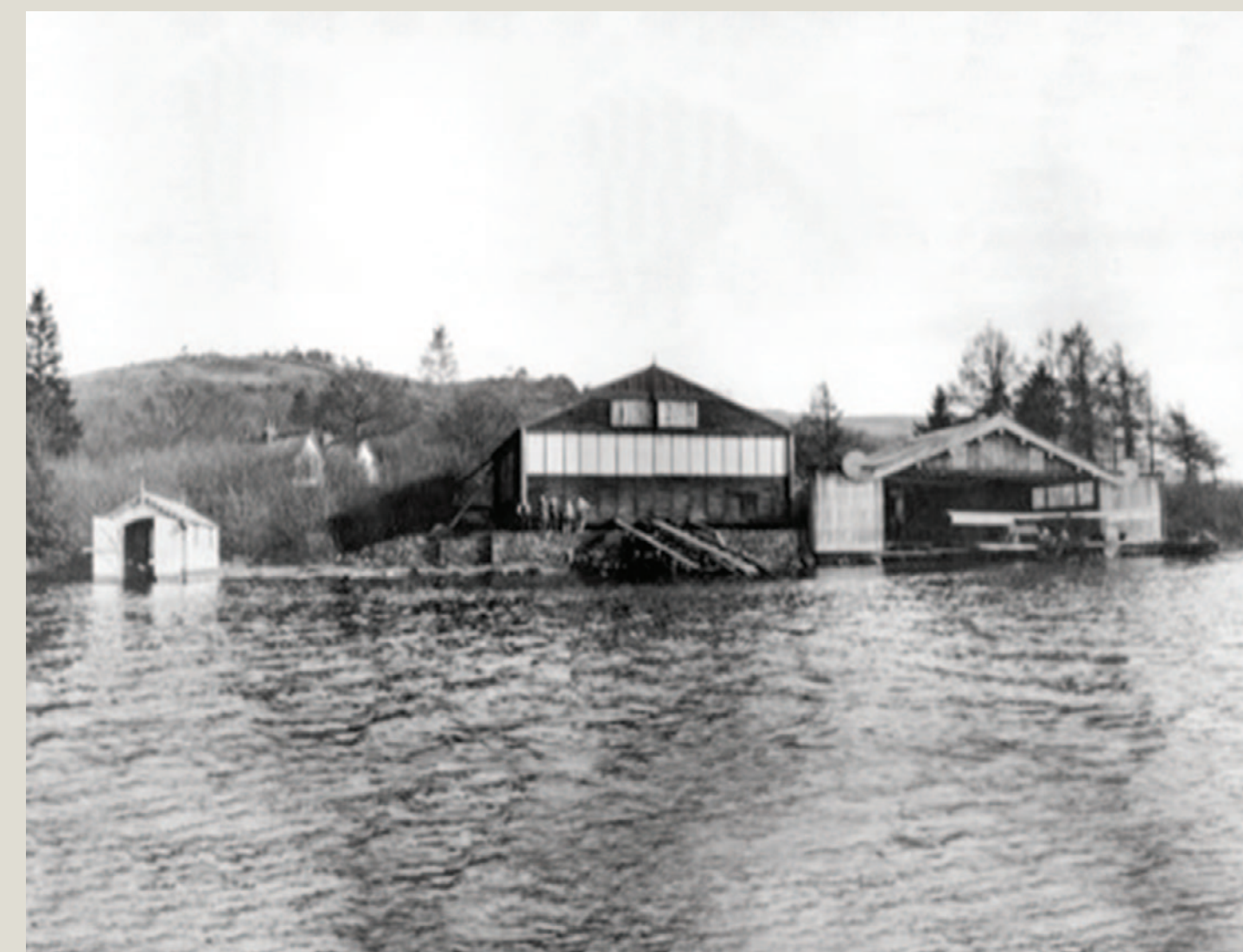
Hangars at Hill of Oaks
