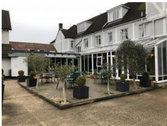
Rear Access from car park to reception, bar, restaurant & conference room
